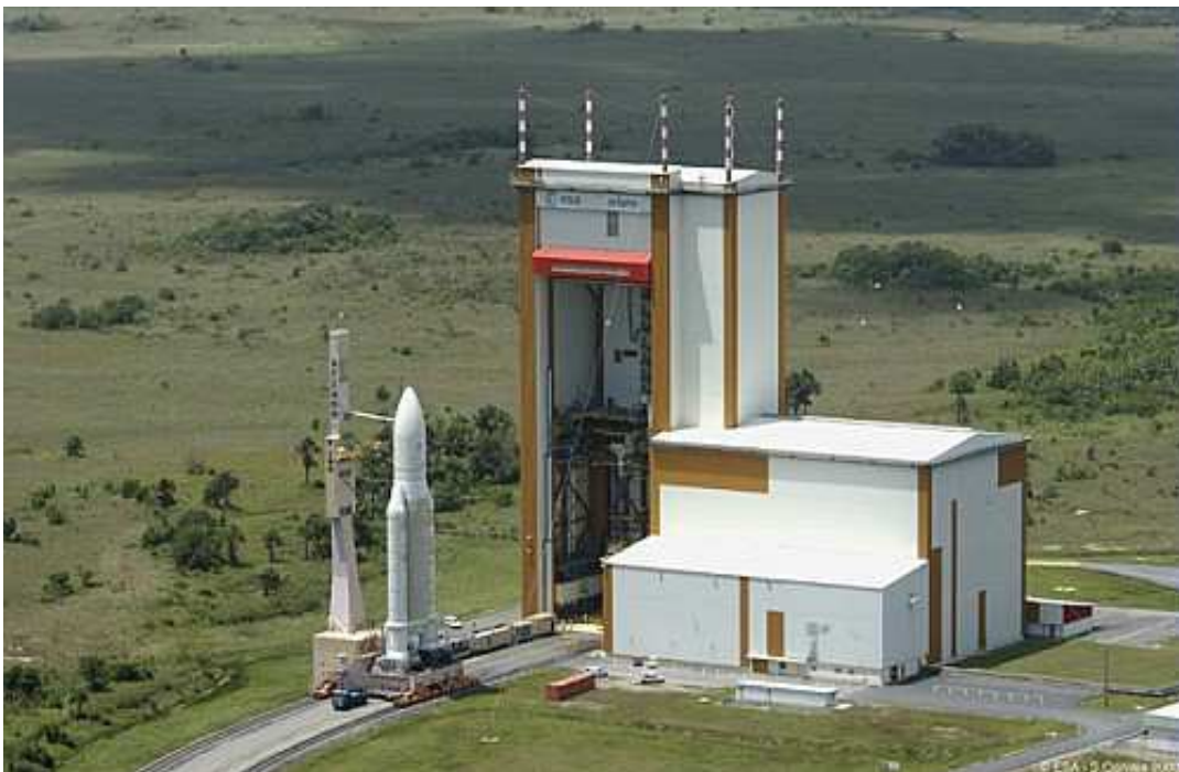
Figure 6.2.3.1.1.a – BAF launch vehicle access side
